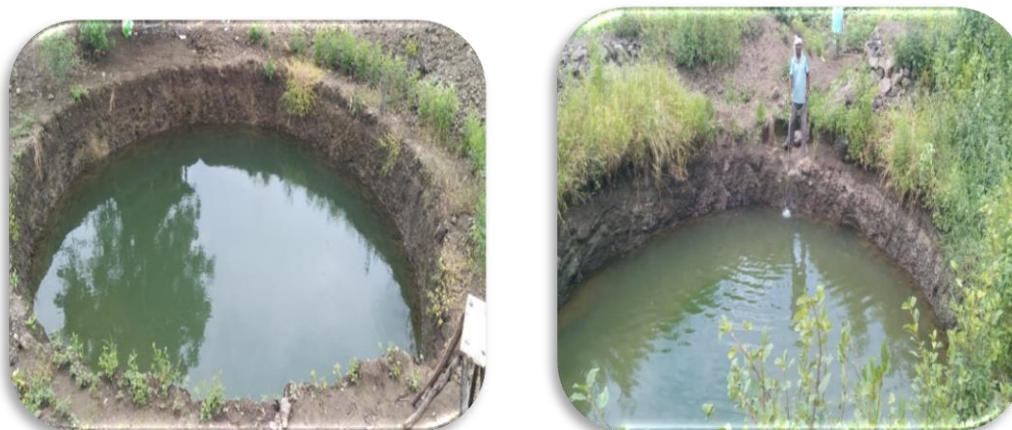
Constructed Recharge Pits filled with Water
